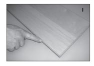
order to use the tongue/groove system. Lay the first row along the wall (note that an expansion/contraction area of minimum 1/2" (12mm) must be provided at the wall, as well as at all columns, heating pipes, doorframes, etc.)
