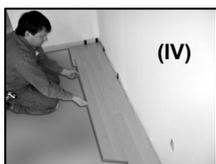
Do not attempt to knock the Uniclic® joint into place with one hit. Continue this method for each plank, covering the entire width of the room.
