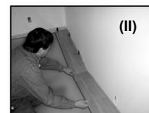
Ensure that the planks of the first row are straight (III). The cut piece from the first row becomes the starting piece for the second row. Install the cut edge facing the wall, with the expansion wedge in place. Now angle this piece and click it into the first plank of the first row.
