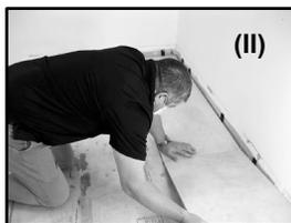
The cut piece from the first row may need to be cut to become the starting piece for another row. The cut pieces should be a minimum of 8" (20 cm) in length.
