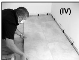
**If necessary, lightly tap both the long and short sides to make sure the pieces are fully engaged. Repeat, until the row is complete.**
